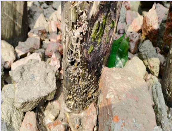
Tubes attached to a broken pole
